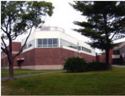
Engineering & Science Research Building, University of Maine, Orono, Maine
