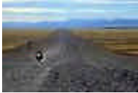
Unpaved Dirt Roads
