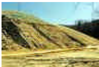
Slopes, Berms & Banks
