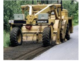
Recycled Asphalt Road Dust Control Road Reclamation Milling Stabilization
