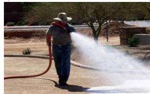
Standard Hose & Pump Hand Spraying
